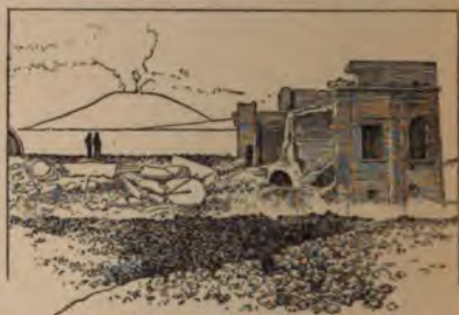
FIG. 140.—One of the villas in Boscotrecase which was ruined by the Vesuvian lava flow of 1906. The fragments of masonry from the ruined walls traveled upon the lava current, where they sometimes became incased in lava.
